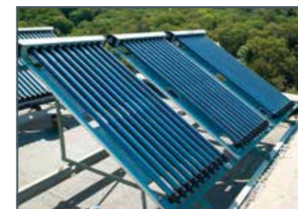
Tube collectors mounted at an optimised angle of incidence on a flat roof
